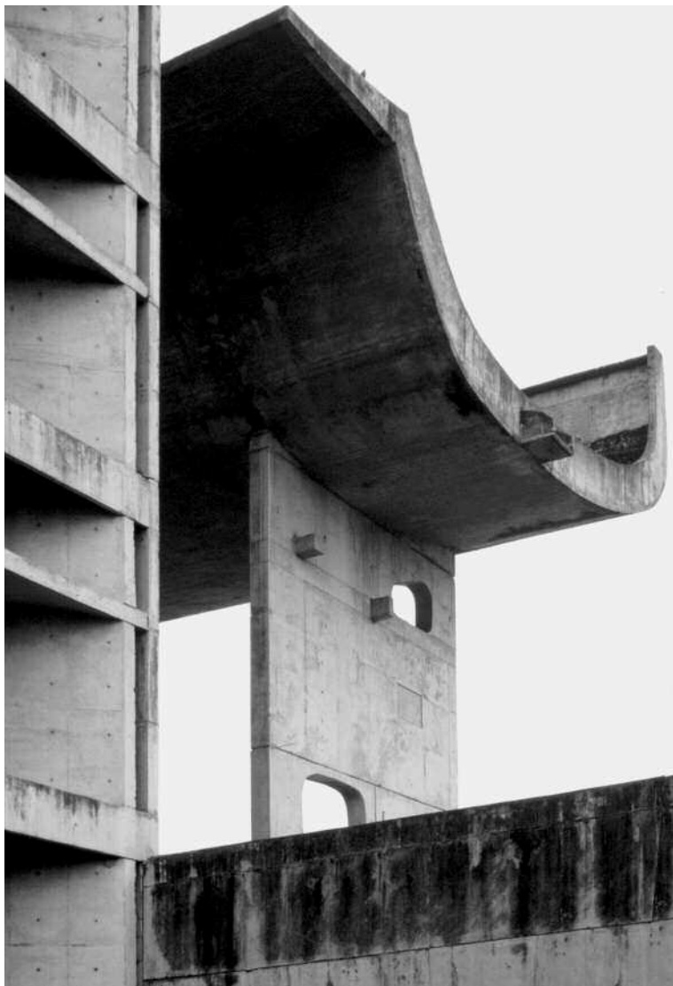
Le Corbusier, Legislative Assembly, Chandigarh, 1955–60, detail of entrance canopy.
