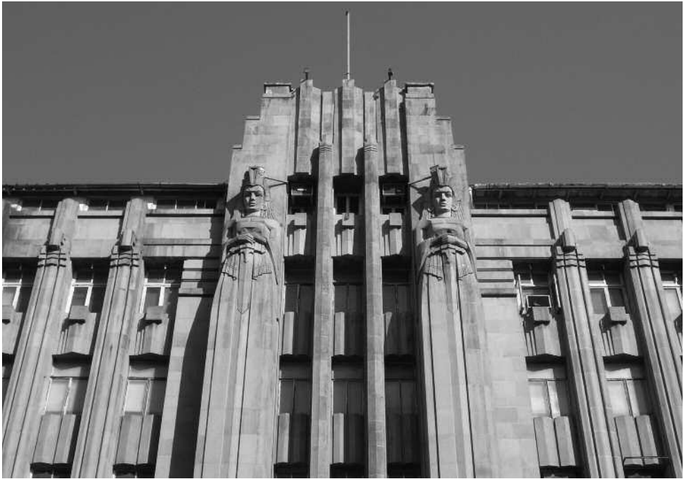
Master, Sathe & Bhuta, New India Assurance Building, Bombay, 1935, facade detail.
