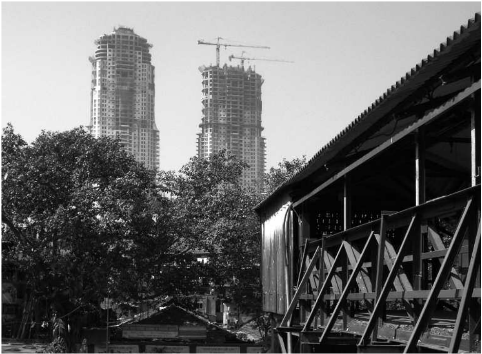
Hafeez Contractor, The Imperial residential condominium towers under construction in Mumbai in early 2008.
