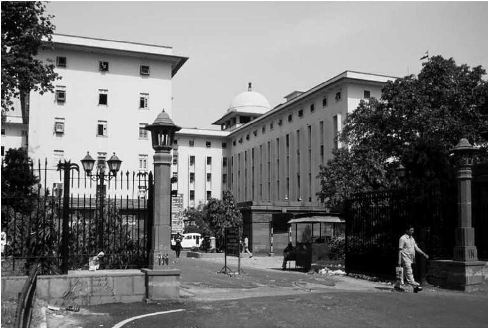
Central Public Works Department, Udyog Bhawan, office block for Ministry of Commerce and Industry, New Delhi, 1957.
