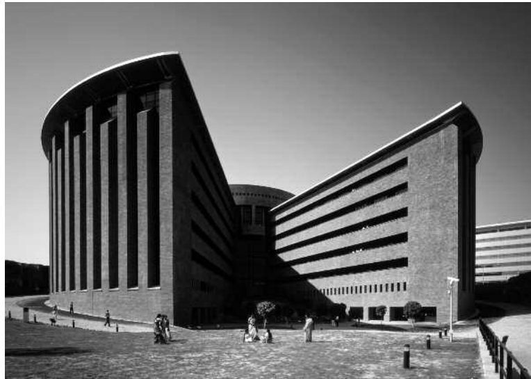
Mario Botta, office block for Tata Consultancy Services, Hyderabad, 2003.
