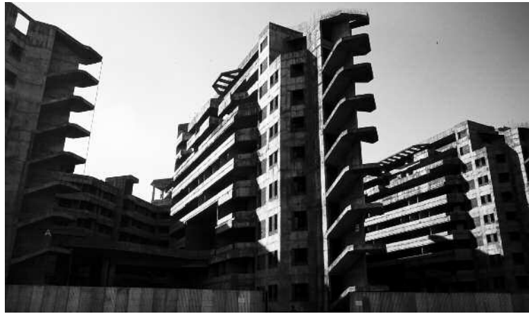
B. V. Doshi and associates, Bharat Diamond Bourse, Mumbai, 1993–7, view and plan of partially constructed scheme.
