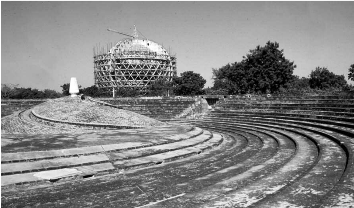
Roger Anger, Matrimandir, Auroville, Tamil Nadu, 1970–2008, concrete superstructure under construction in 1985.
