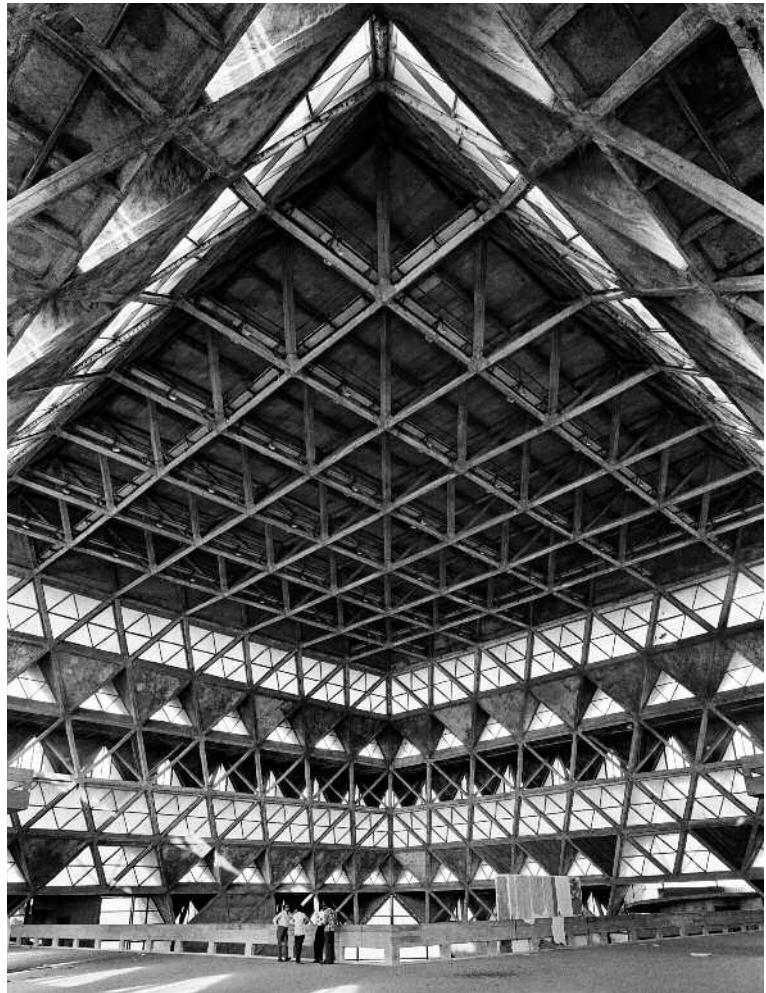
above and right: Raj Rewal, permanent exhibition structures at Pragati Maidan, New Delhi, 1971–2, under construction in late 1972, and interior view.
