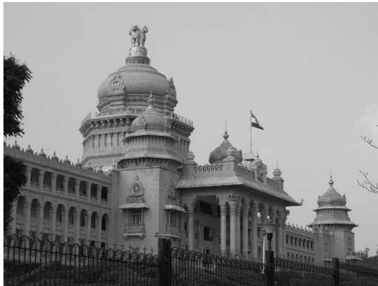
B. R. Manickam and Karnataka Public Works Department, Vidhana Soudha, State Legislative Assembly Building, Bangalore, 1952–7.
