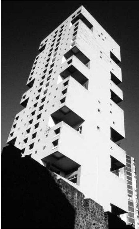
Charles Correa and Pravina Mehta, Kanchanjunga Apartments, Bombay, 1970–83.
