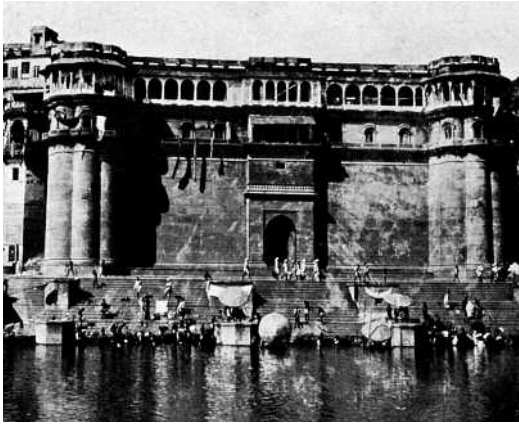
Modern ghats at Benares constructed in the late 19th century, photographed by Gordon Sanderson of the Archaeological Survey of India and first published in 1913.
