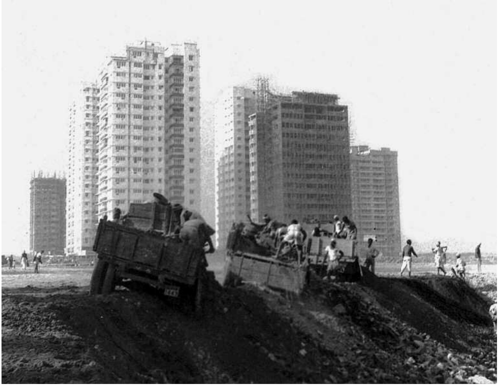
Back Bay land reclamation work in progress, Bombay, 1970s.
