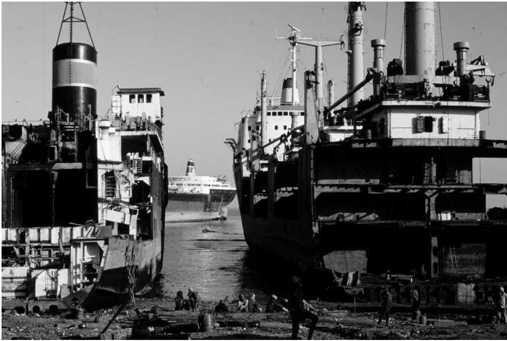
Ship-breaking at Alung, Gujarat, 1986.
