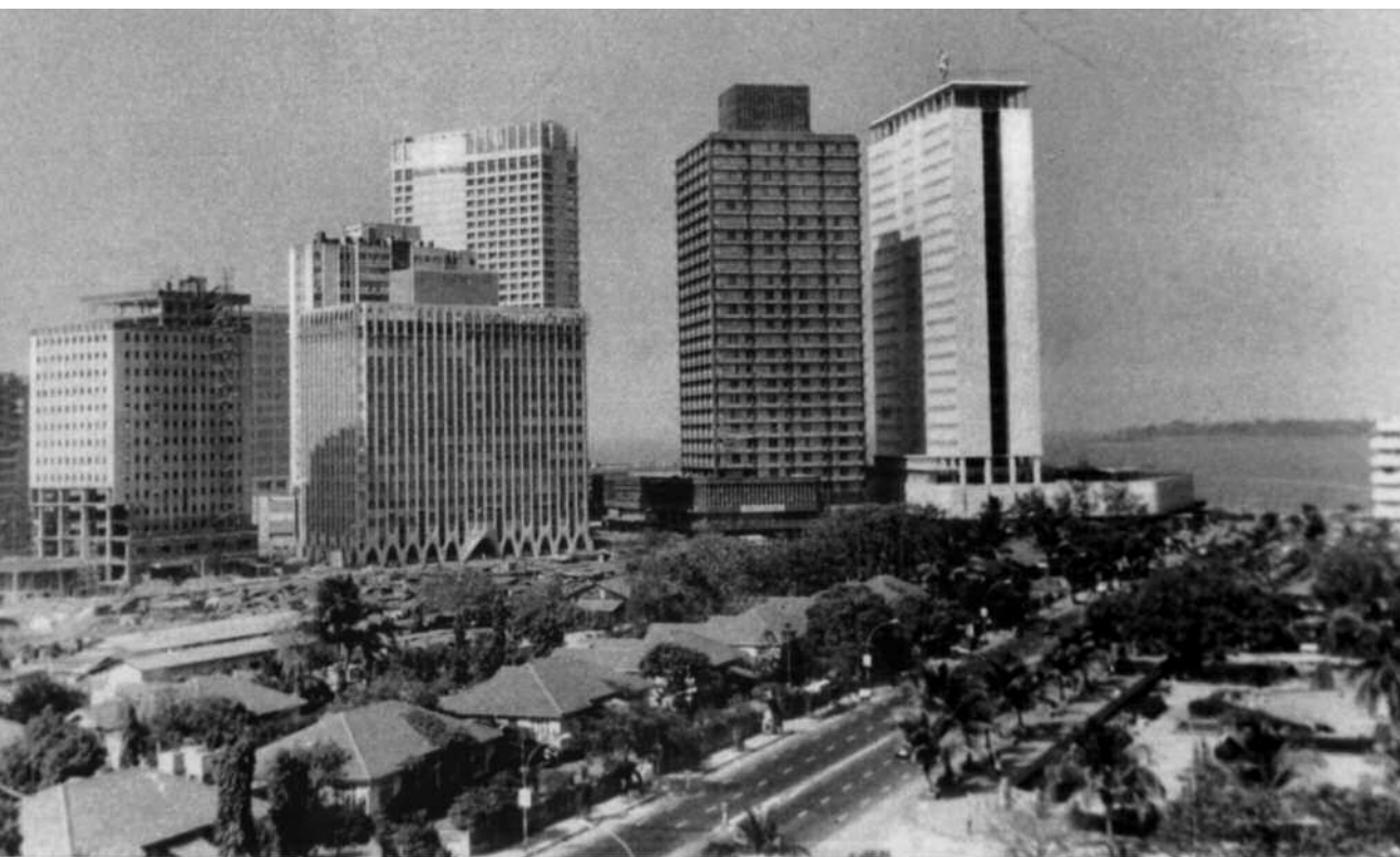
Air India Building and other high-rise office buildings under construction at Nariman Point, Bombay, mid-1970s.
