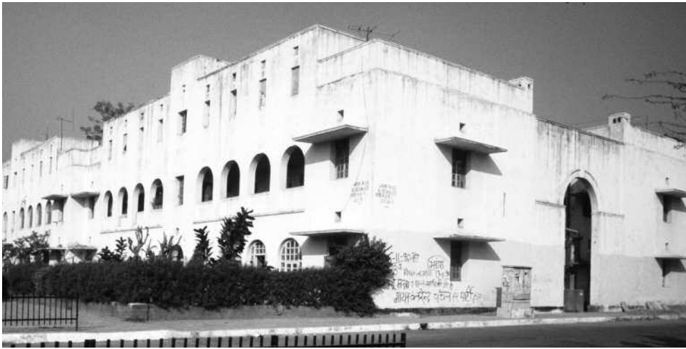
Central Public Works Department, Government Officers' Flats at Lodi Colony, New Delhi, late 1940s.
