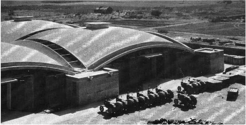
Joseph A. Stein & Associates, Escorts Industrial Campus, Faridabad, Uttar Pradesh, 1960–88, concrete shells for storage facilities and interior view, 1965.
