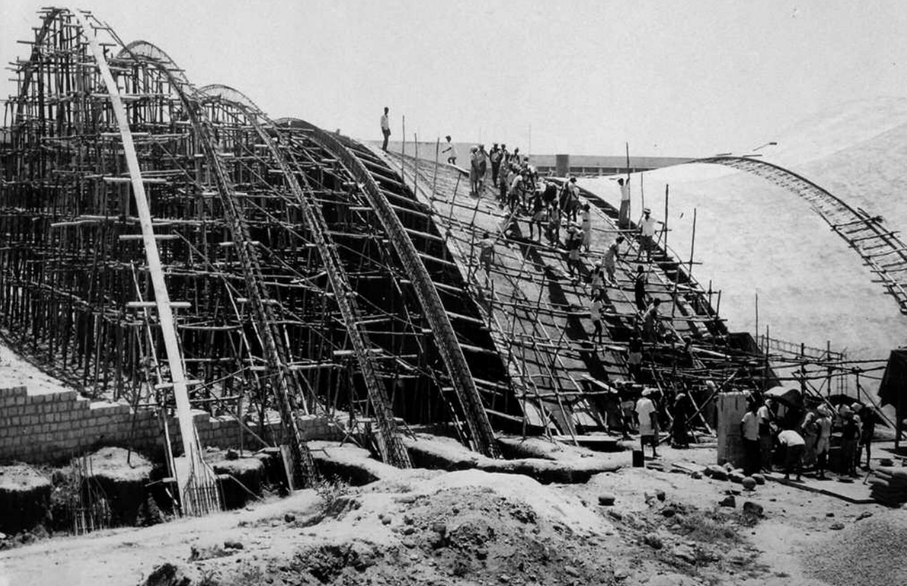
S. L. Chitale, Auditorium at Sri Venkateswara University, Tirupati, Andhra Pradesh, 1970–75, hyperbolic paraboloid roof under construction.
