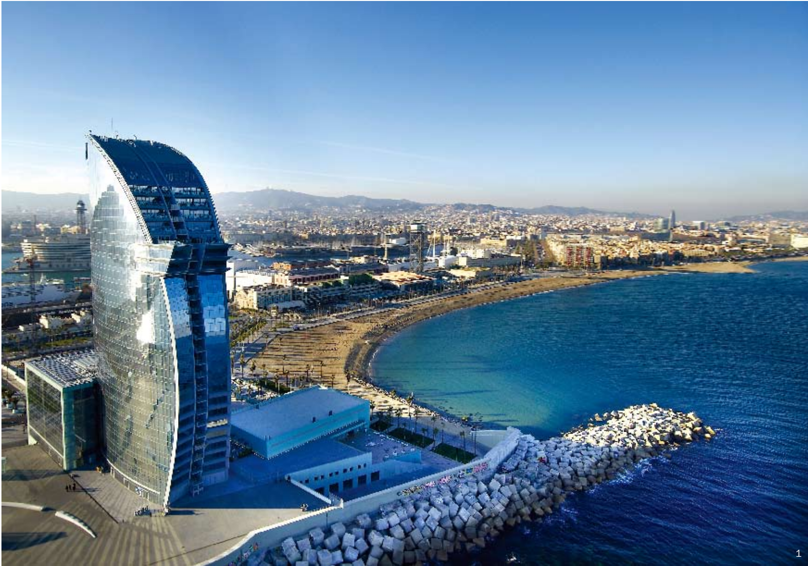
1. General view and background 2. Rooftop bar overlooking the beautiful sea 3. Lounge
