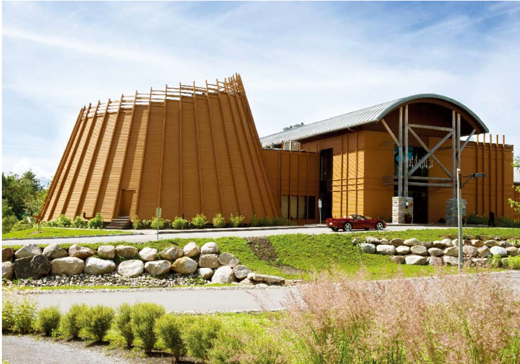
1. Façade facing the road 2. Reclaimed stream in front of the building 3. Grand lobby
