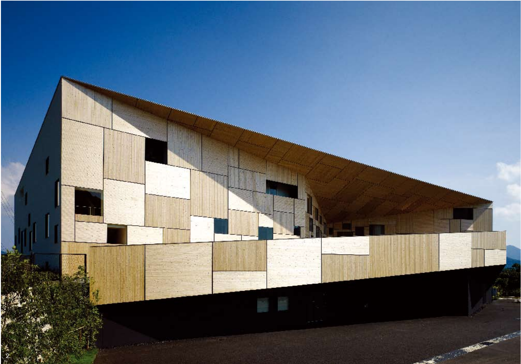
1. North façade 2. East façade 3. West façade
