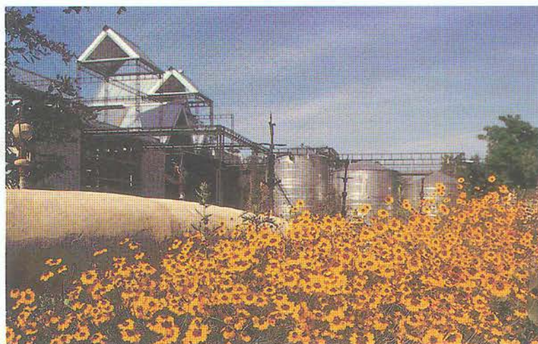
The Advanced Green Builder Demonstration CMPBS Austin, Texas, USA 1994-97
