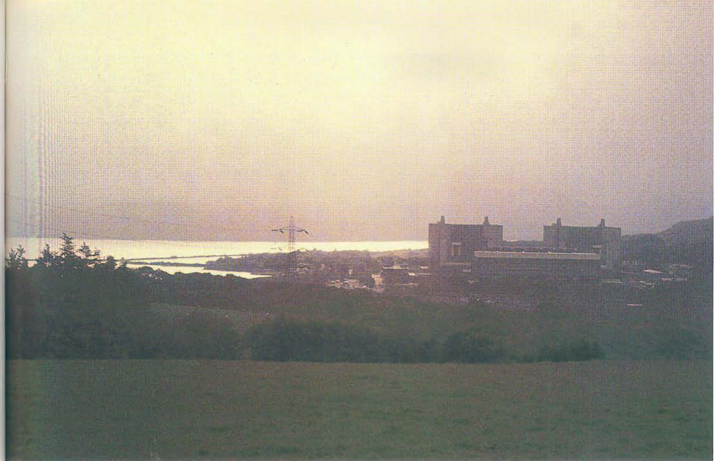
Nuclear Power Station Sir Basil Spence Trawsfynydd, Wales 1959
