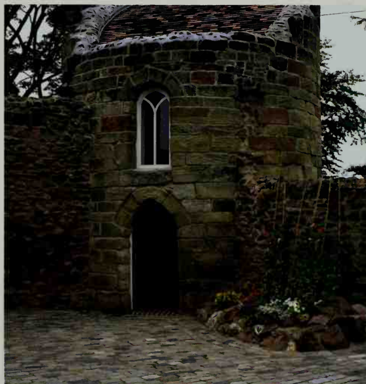
Below: Three shorter towers, one shown here, were used for a larder, bakehouse, and stables.
