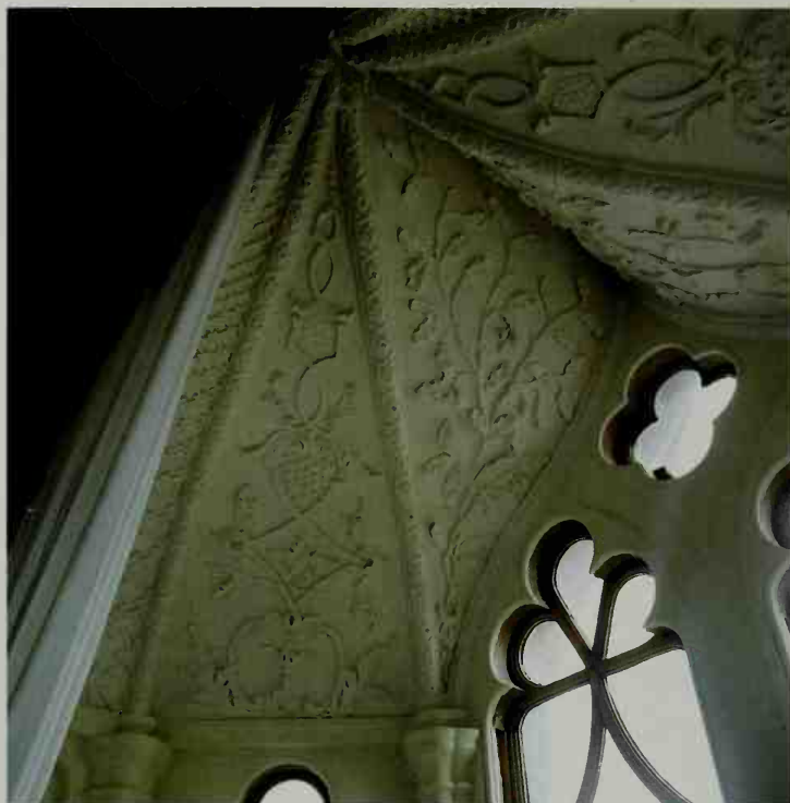
A detail of one of the Gothick windows in the blue drawing room highlights the outstanding craftsmanship of the lovely plasterwork. The oak branch is a typical early Gothic motif.
