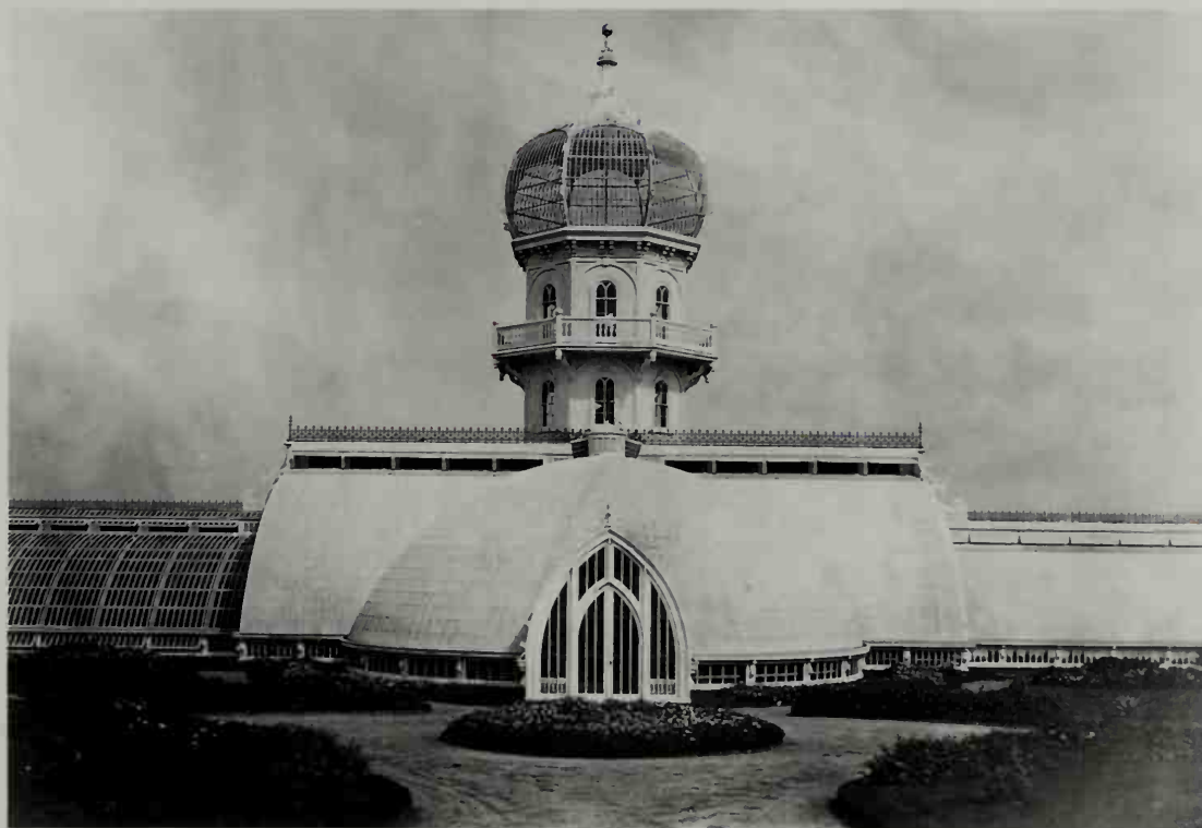
The first greenhouse was built on the Lyndhurst estate about 1870 by George Merritt. It was wonderfully fanciful, with an enormous onion-dome top.
