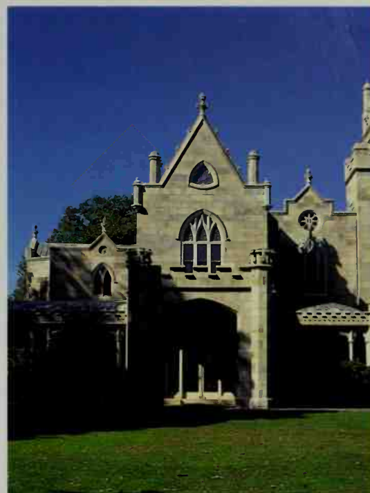
During remodeling, the original porte cochère was enclosed in glass and transformed into a vestibule with a veranda extending from either side. A new single-story turreted porte cochère was built in front of it.
