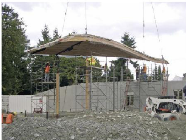
Perkins+Will Canada, VanDusen Botanical Garden Visitor Centre, Vancouver, 2011 The Glulam roof panels for VanDusen were prefabricated approximately 40 kilometres (25 miles) away and installed on site.
