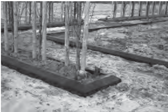
The construction of the border of the soccer field
