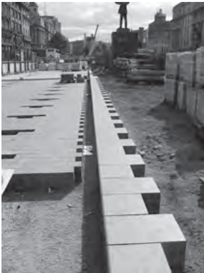
2.14 Construction of granite kerb and carriageway paving 2.15 Details at the base of the Spire, including protective bollards
