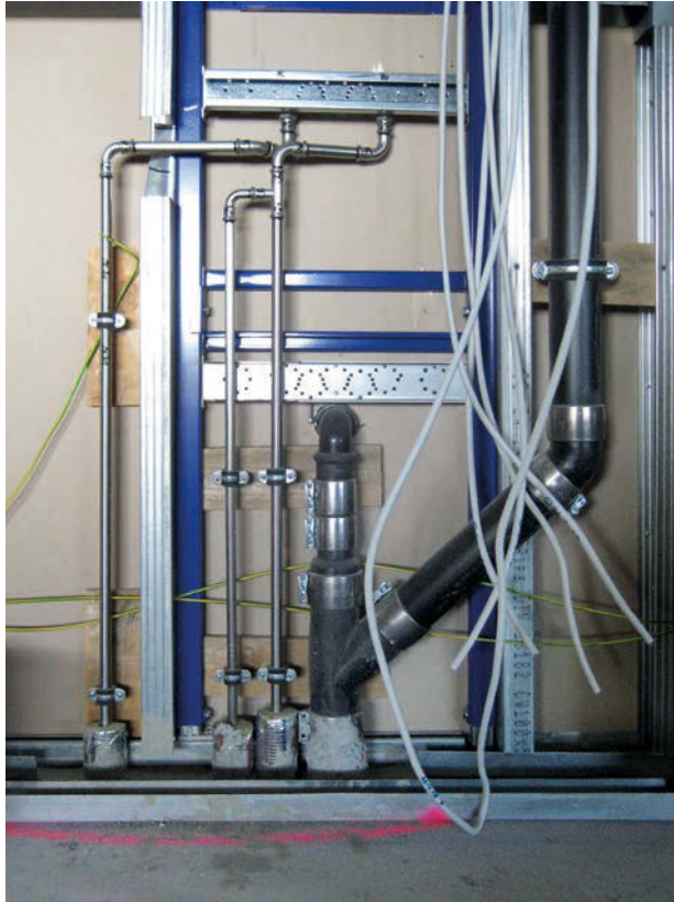
Mounting and utility connections for a washbasin in a plasterboard wall duct.
